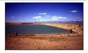
Figure 3. Earth embankment to retain rainwater for groundwater recharge in Iran
