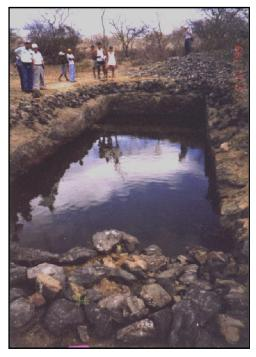
Figure 2. Excavation work to construct a rock catchment in Brazil
