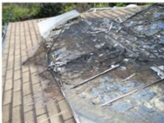
Figure 9. Fire in PV Solar Panels due to an Electrical Arc
