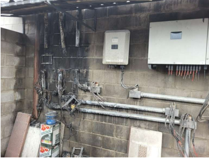
Figure 8. Fire in a solar energy system
